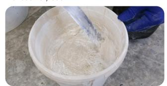
**Step Seven**Optionally, create chopped strand reinforced premix and apply for further stability.
