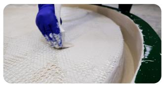
**Step Five**Wet with mix and apply Quadaxial Glass Fabric into touch dry coat.
