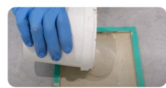
**Step Seven**Back-fill with AC630/730/830 solid/laminated.
